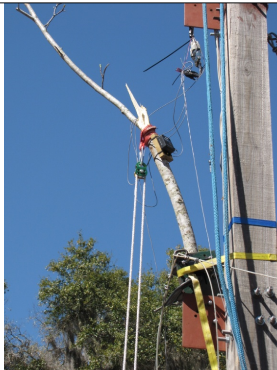
Vertically oriented branches typically failed beyond the first pulley at or near a branch union.
